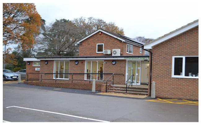
Reside Construction Limited has successfully completed an extension of Finchampstead Surgery in Wokingham, Surrey. The premises are currently in use as a large primary care surgery and were built in the 1970s with traditional brick and pitched roof covering the ground and first floor.
